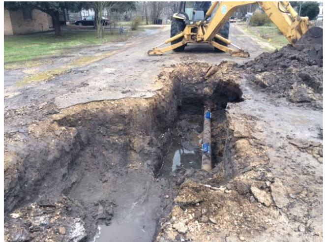
*City Crew fix a 6" main water line on Colfax Street. The line was fixed "Hot" meaning under high pressure.*
